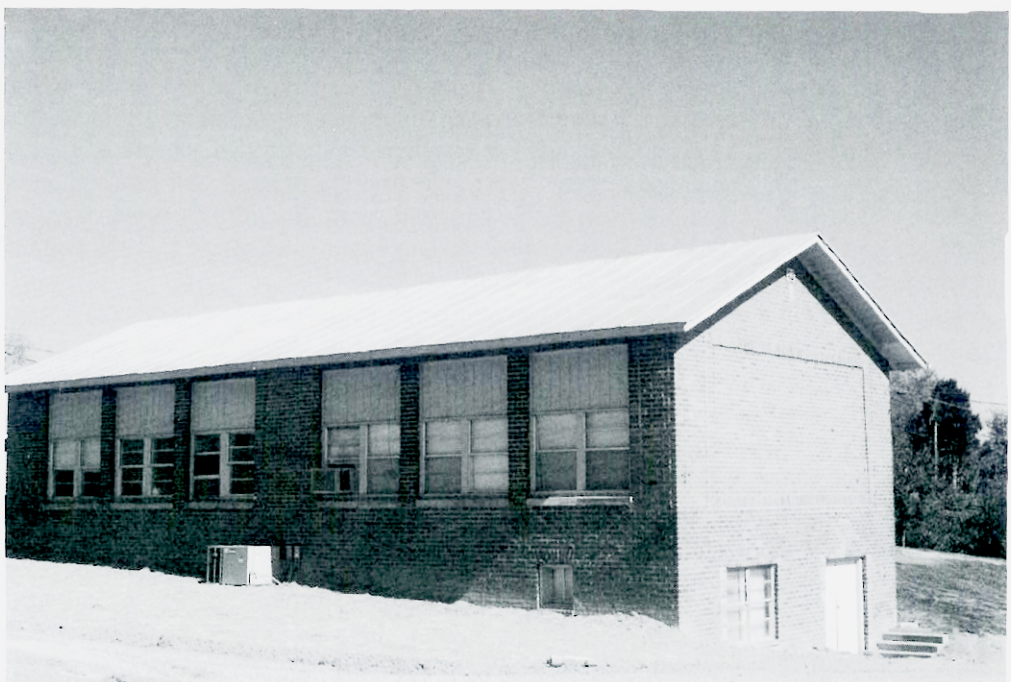
Figure 1-54. The rear facade of the Pleasant View Rosenwald School, which was built by the J, F & N McMahan Construction Company with donated labor and materials.
